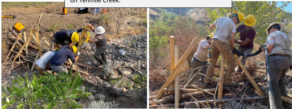
Conservation Corps using a post pounder to install PALS on Tenmile Creek.
