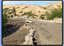
The fish passage barrier had limited access to spawning and rearing habitat for native salmonids, including Endangered Species Actlisted (ESA) Steelhead within Cottonwood Creek. The existing culvert was removed and replaced with a three-sided concrete box culvert on
