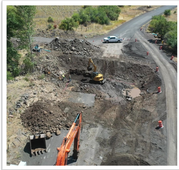
Construction on Cougar Creek fish passage
