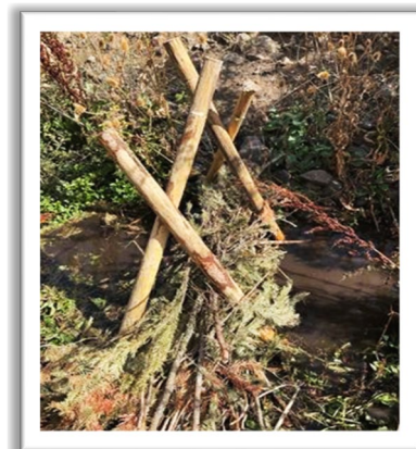
New BDA (beaver dam analog) & PALS (post assisted log structure) on Kelly Creek
