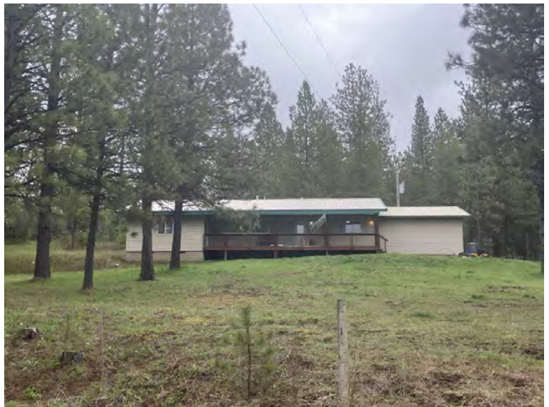
This home in the Anatone Forestland zone has many of the recommended home hardening and defensible space measures completed. Photo credit: The Ember Alliance.
