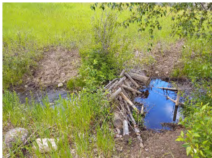
Post-assisted log structures can increase the ability of streams to capture sediment and increase the resilience of riparian areas to wildfire.
