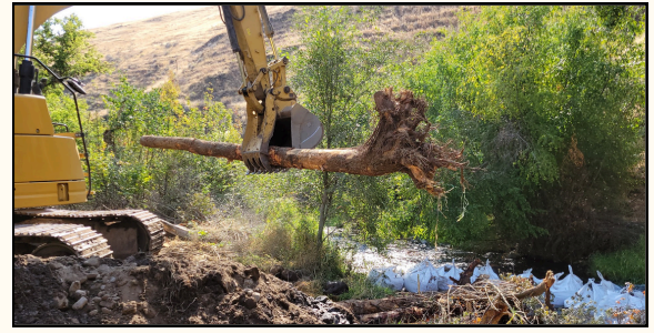
Above Image: Excavator building Steelhead Habitat
