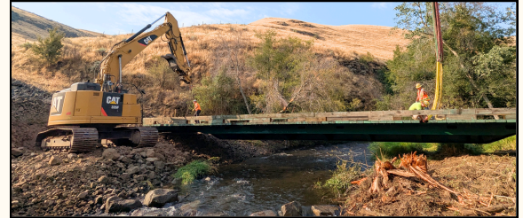
Above Image: Livestock Crossing Bridge
